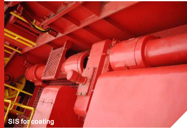
Electric control cabinet
